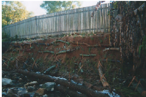
Erosion control along Burnt Bridge Creek
