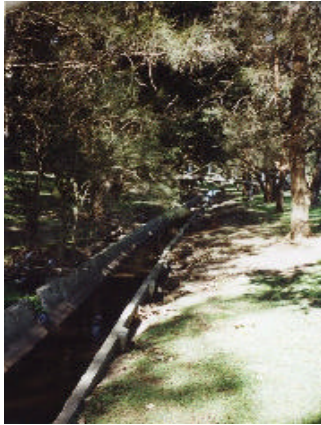
Dee Why Creek concrete channel below Cambell Avenue
