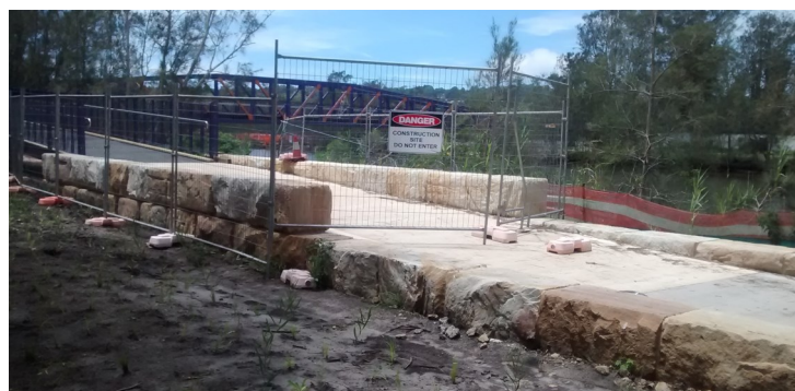
Approach to bridge north of Middle Creek is in place.
