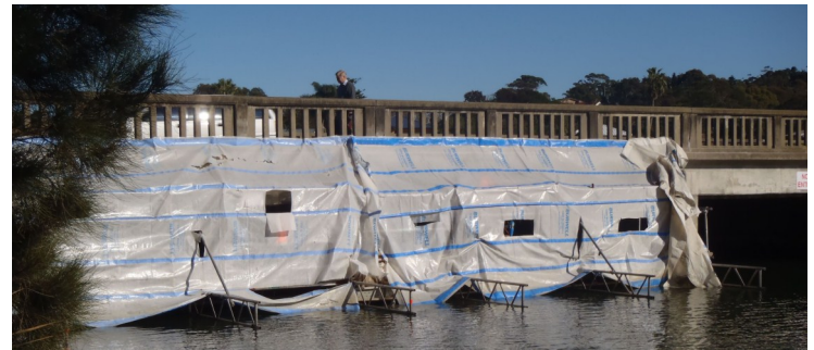
Bridge over Narrabeen Lagoon being repaired but not widened
