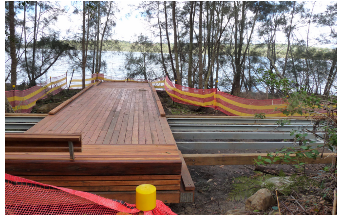
Viewing platform in Stage 1 of Lagoon Walkway
