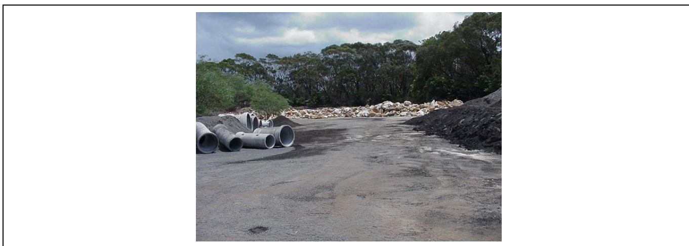
Photo 31: The former quarry now used to store construction materials within Lot 1334.
